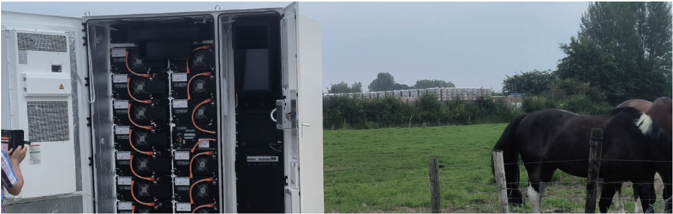
• The Netherlands 100kW/215kWh DH200F PV consumption (self-use)
