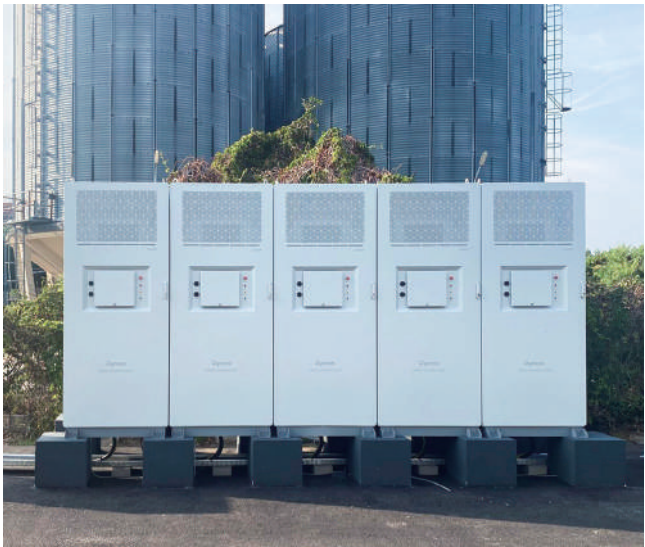
• Spain 500kW/1160kWh DH200Y Self-generation and self-use+PV consumption
