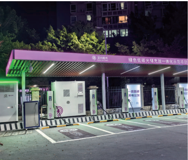
• China 100kW/215kWh DH200F Peak-to-valley arbitrage + Dynamic capacity increase
