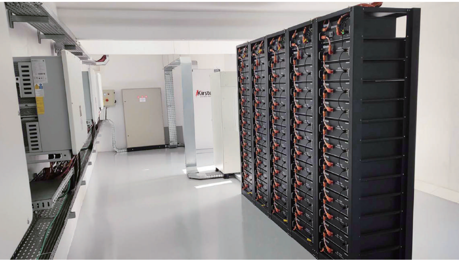
• Brazil 100kW/307kWh PowerRack HV4F Dynamic capacity expansion (peak-shaving) + PV consumption
